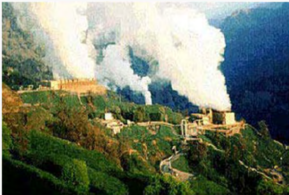
Geothermal Power Plant
