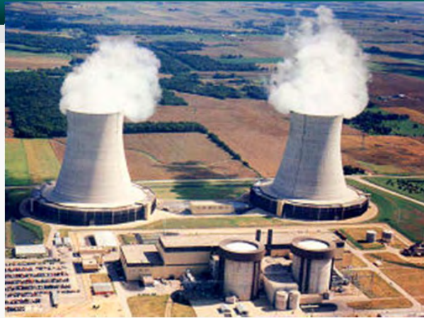
Nuclear Power Plant
