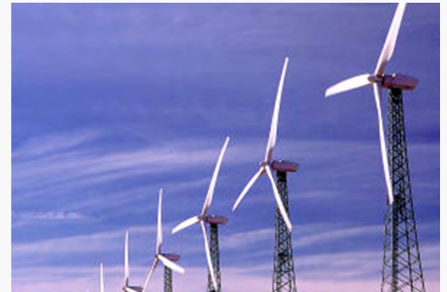
Wind Power Towers
