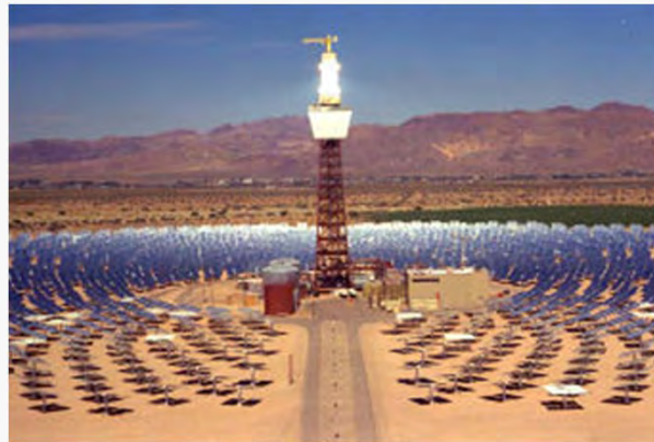
Solar Thermal Power Plant
