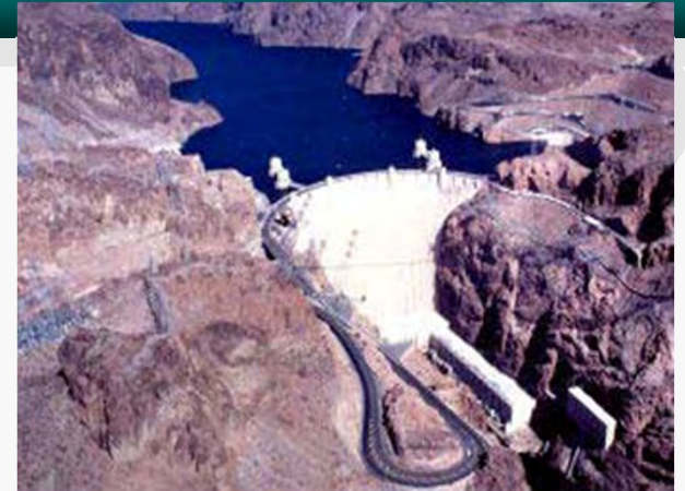
Hydroelectric Power Plant
