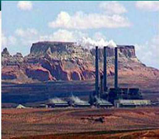
Fossil Fuel Power Plant
